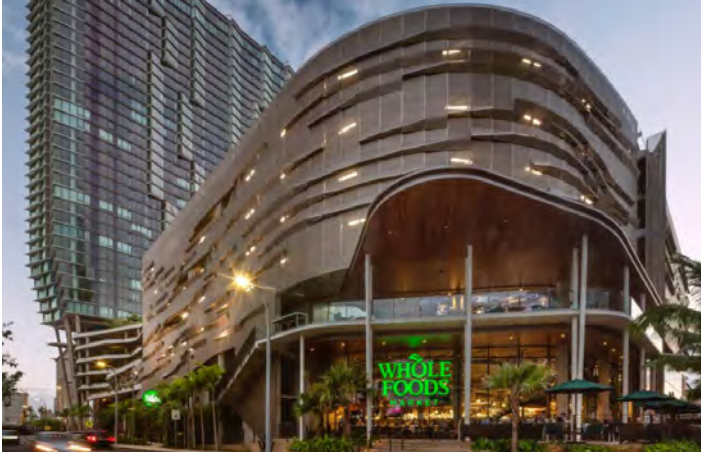
Project: A'eo Tower, Honolulu. Source: www.wardvillage.com
