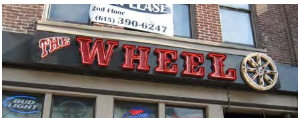
Example of raceway incorporated as sign background
