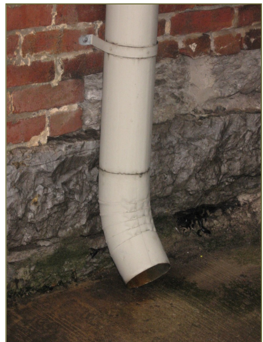
Downspouts should channel water away from the building foundation.
