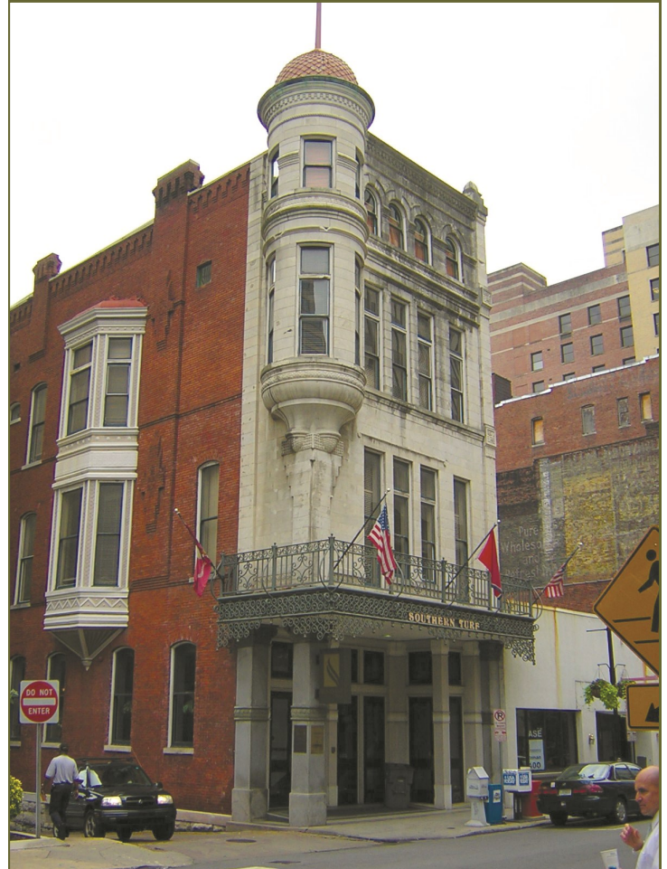
Character-defining features of the building at 224 Fourth Avenue include the corner turret, side bay window and metal canopy.
