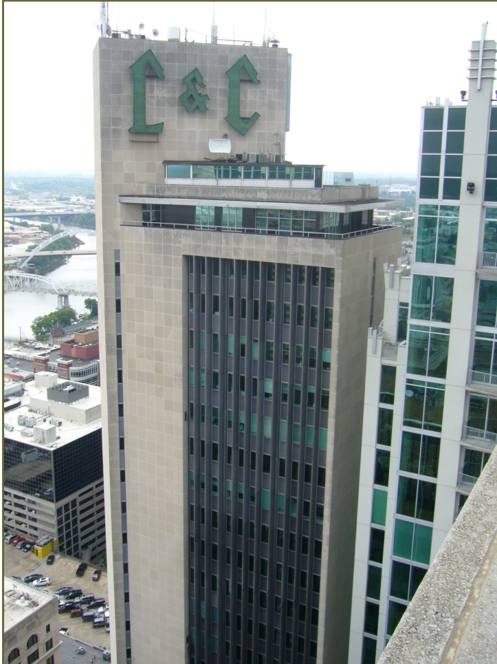
Roofs in the district are primarily flat or appear to be flat with a parapet wall.
