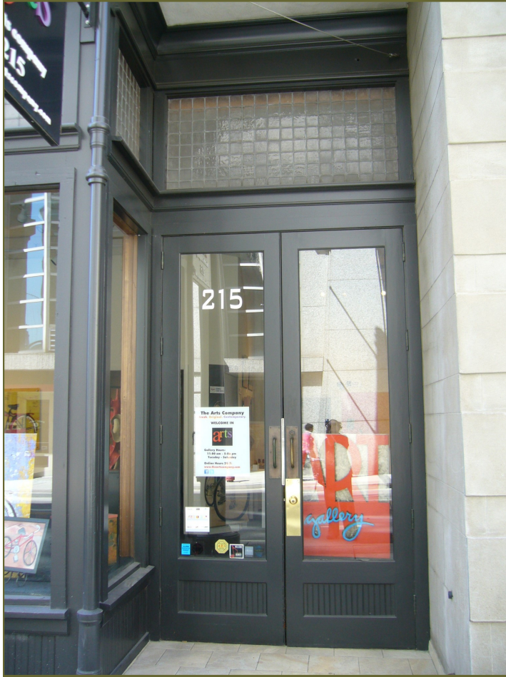
Historic transoms above windows and doors should be retained and preserved.
