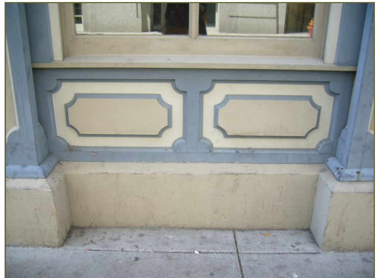
The painted, paneled wood is an appropriate modern bulkhead design.
