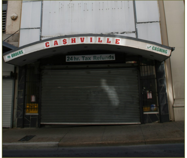
The original storefront has been removed; however, the building retains its early arched canopy.
