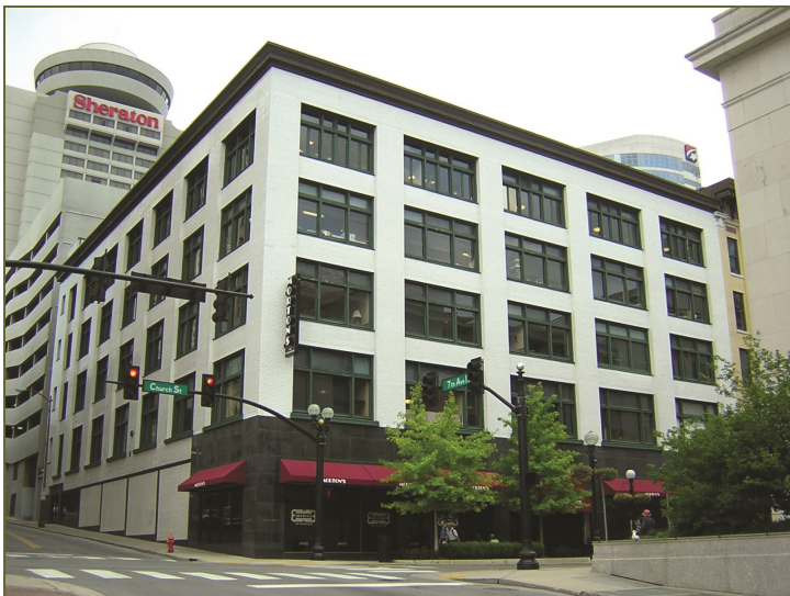
The placement, above the storefront and transom, and shed form of these awnings are appropriate. Likewise, its opaque construction material is appropriate. Awnings may include graphics or signage.
