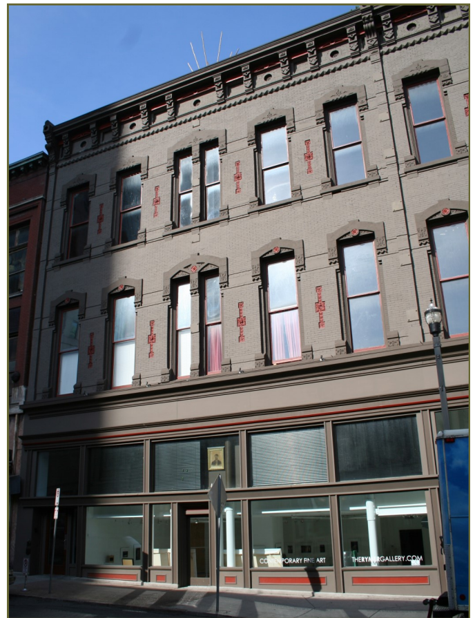
Some storefronts have their own cornices, like this one at 233 Fifth Avenue North. These should also be retained and remain visible.
