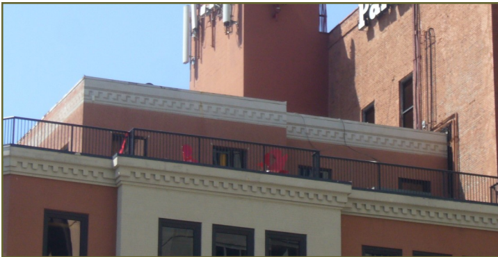
This rooftop addition, constructed prior to the overlay, sits back from the walls below and is only one story tall, making it minimally visible from the street.
