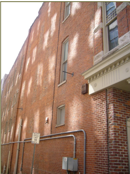
Preserve and maintain historic masonry.
