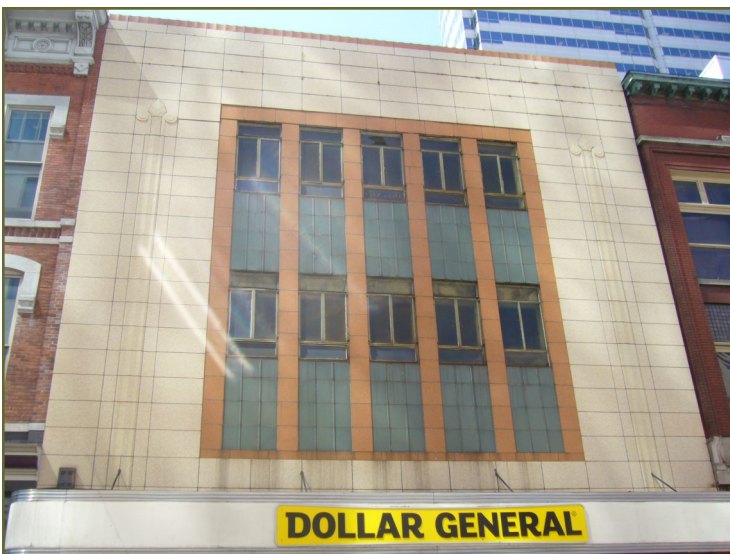
Window styles and materials downtown vary from single and double-hung windows, to metal windows of a more industrial design.
