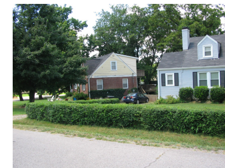
Many of the homes have been expanded by raising the roof on the back of the upper floor.
