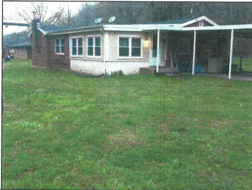
Photo Three Caption LEFT AND REAR VIEW OF RESIDENCE (SOUTHWEST) Clear Photo Three
