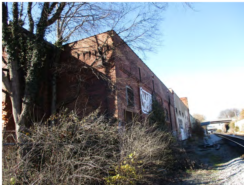
#10 – Rear of Improvement
