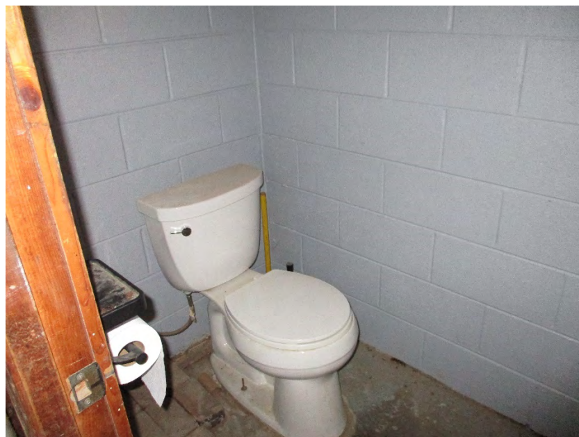
#18 – Interior of Improvement – Restroom
