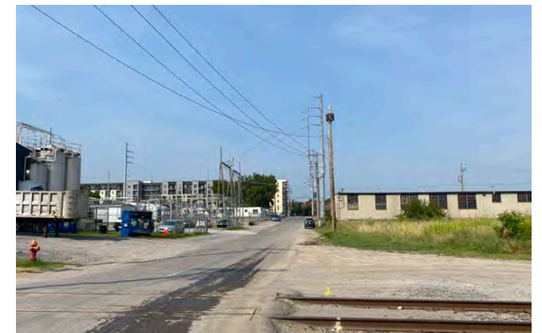
The Van Buren frontage will provide on-street parking, planting zone and 8' sidewalk and will also include a landscaped courtyard to lessen the impact of the NES substation shown.
