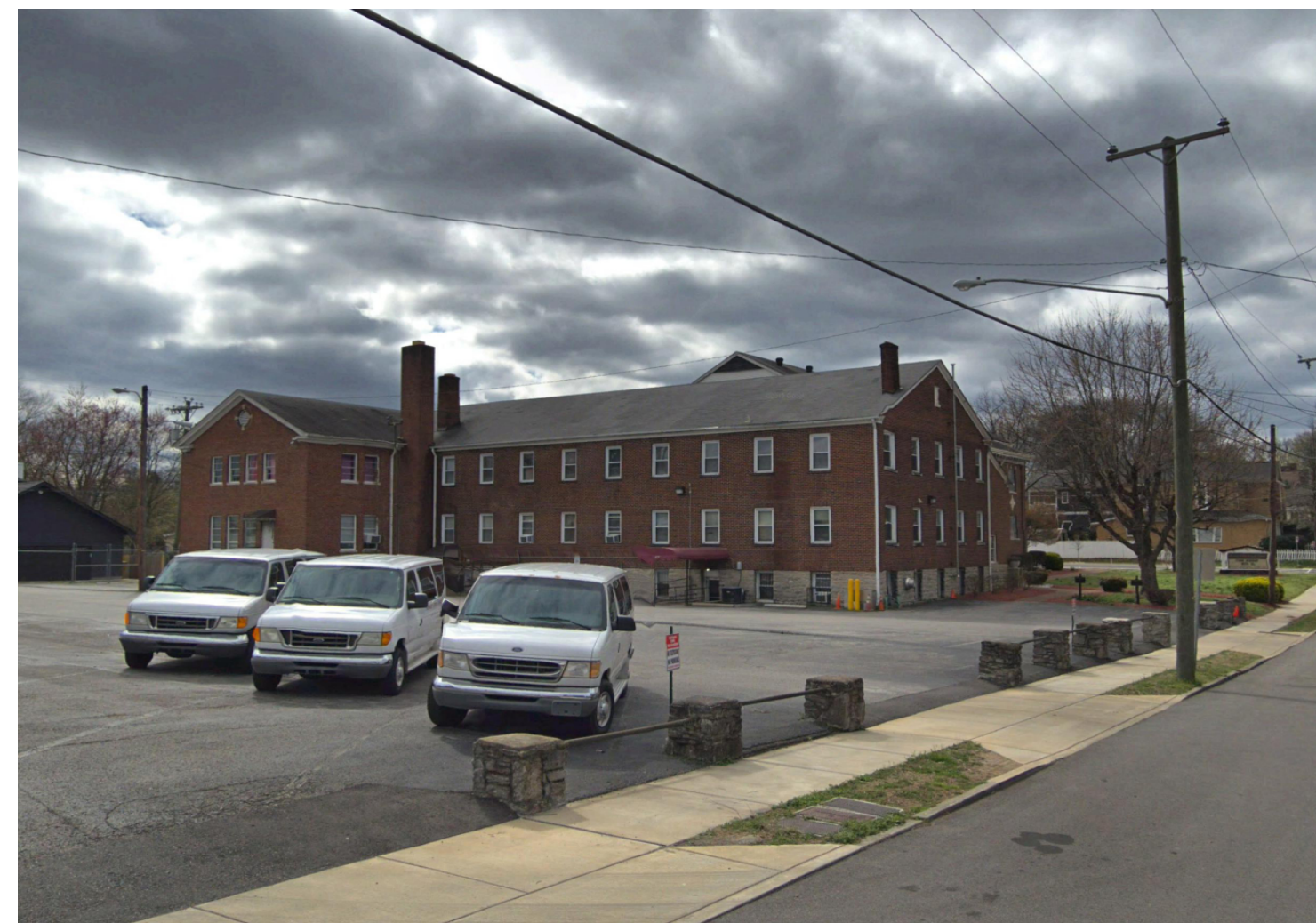
VIEW OF EXISTING BUILDING FROM NORTHEAST CORNER
