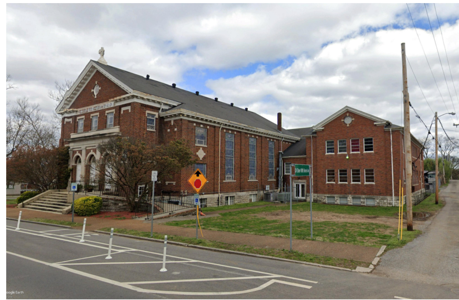
VIEW OF EXISTING BUILDING FROM SOUTHWEST CORNER
