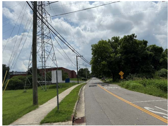
John Mallette Road facing East
