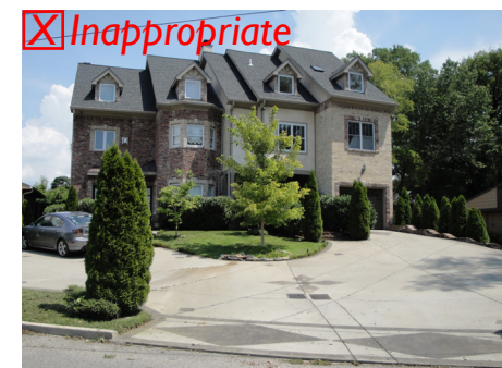
In addition to being too tall, additional parking pads are not permitted in the front yard and driveways are to be 12' maximum.
