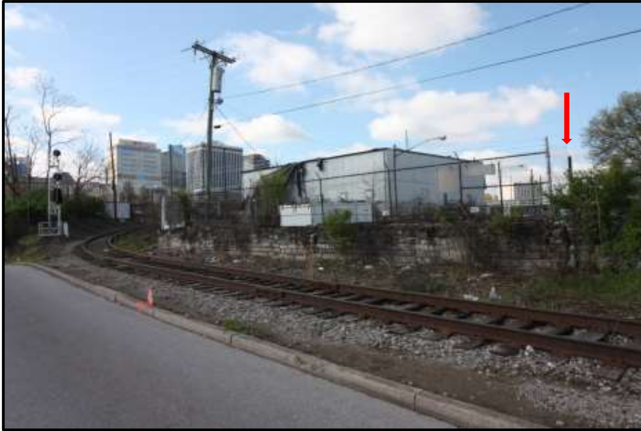
SUBJECT 04/01 /2020 SOUTHEASTERN MOST PROPERTY LINE FOR THE SUBJECT
