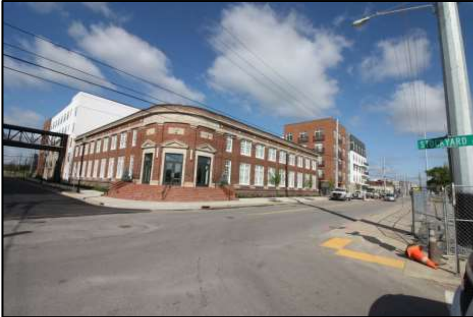
SUBJECT 04/01 /2020 STOCKYARD BUILDING / CORNER OF STOCKYARD STREET AND 2 ND AVENUE NORTH
