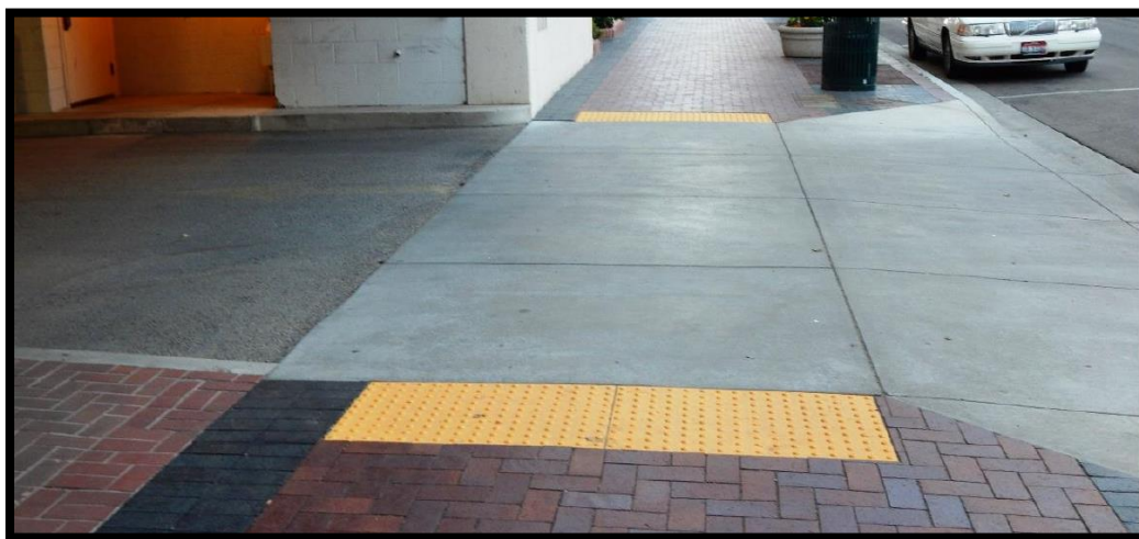
Figure 4-7: Garage Access Ramp Flush with Sidewalk
