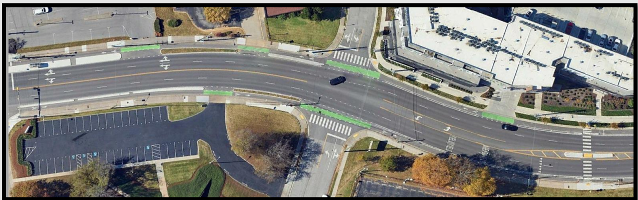
Figure 4-2: Bike Lanes on 12th Avenue South Featuring Green Pavement Markings at Driveway Crossings and Vegetative Buffers (Nashville, TN)
