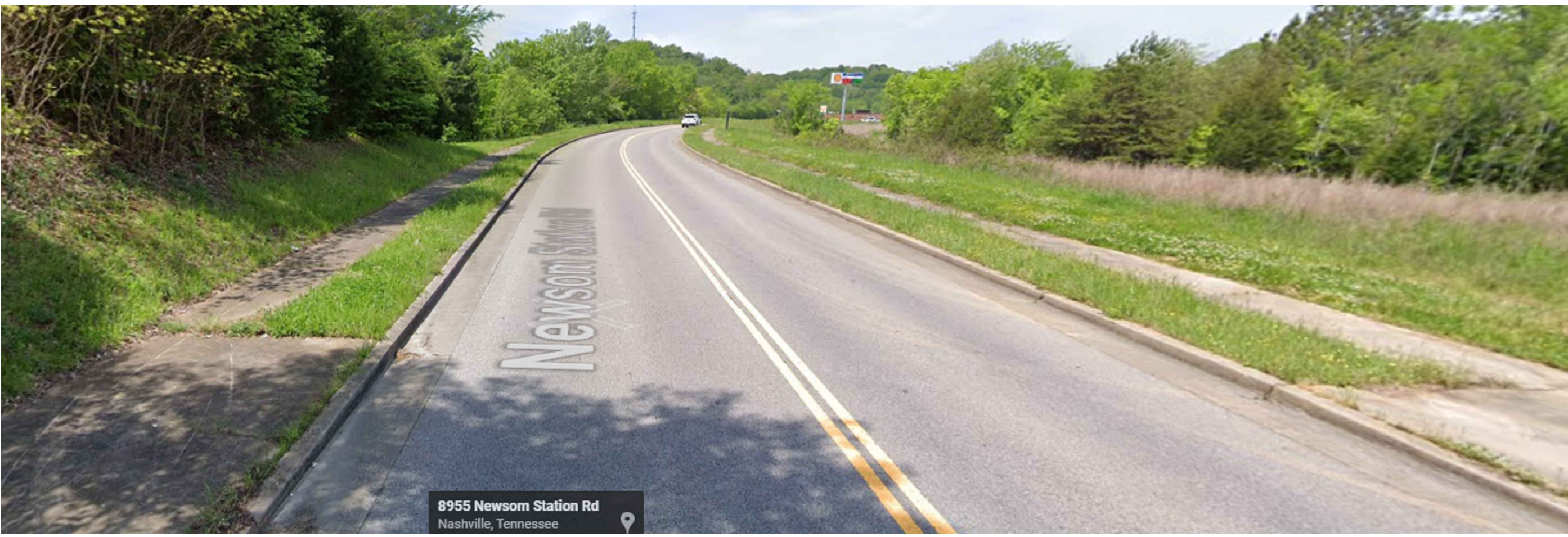
Consolidated Entrance View West - Sight Distance 400 feet +
