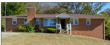
827 Youngs Lane is an example a cantilevered second level.
