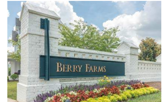
Masonry Signage Wall
