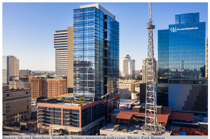
Project: 5th and Broadway, Nashville. Source: www.usa.skanska.com. Photo: Zack Benson
