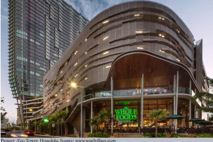
Project: A'eo Tower, Honolulu. Source: www.wardvillage.com
