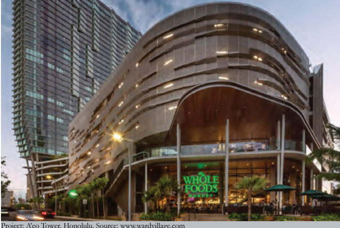
Project: A'eo Tower, Honolulu. Source: www.wardvillage.com
