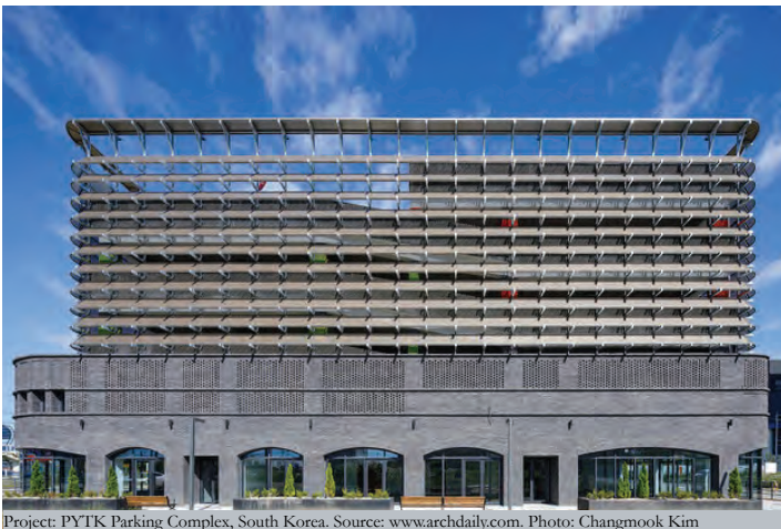
Project: PYTK Parking Complex, South Korea. Source: www.archdaily.com. Photo: Changmook Kim
