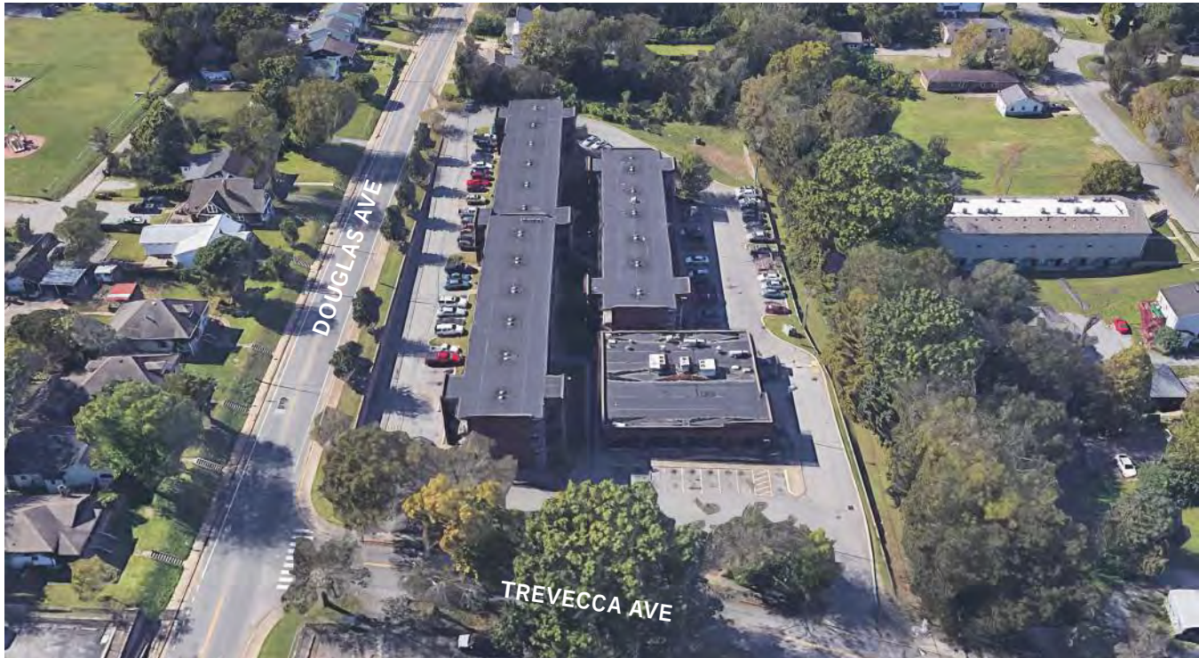
BIRD'S EYE VIEW LOOKING WEST
