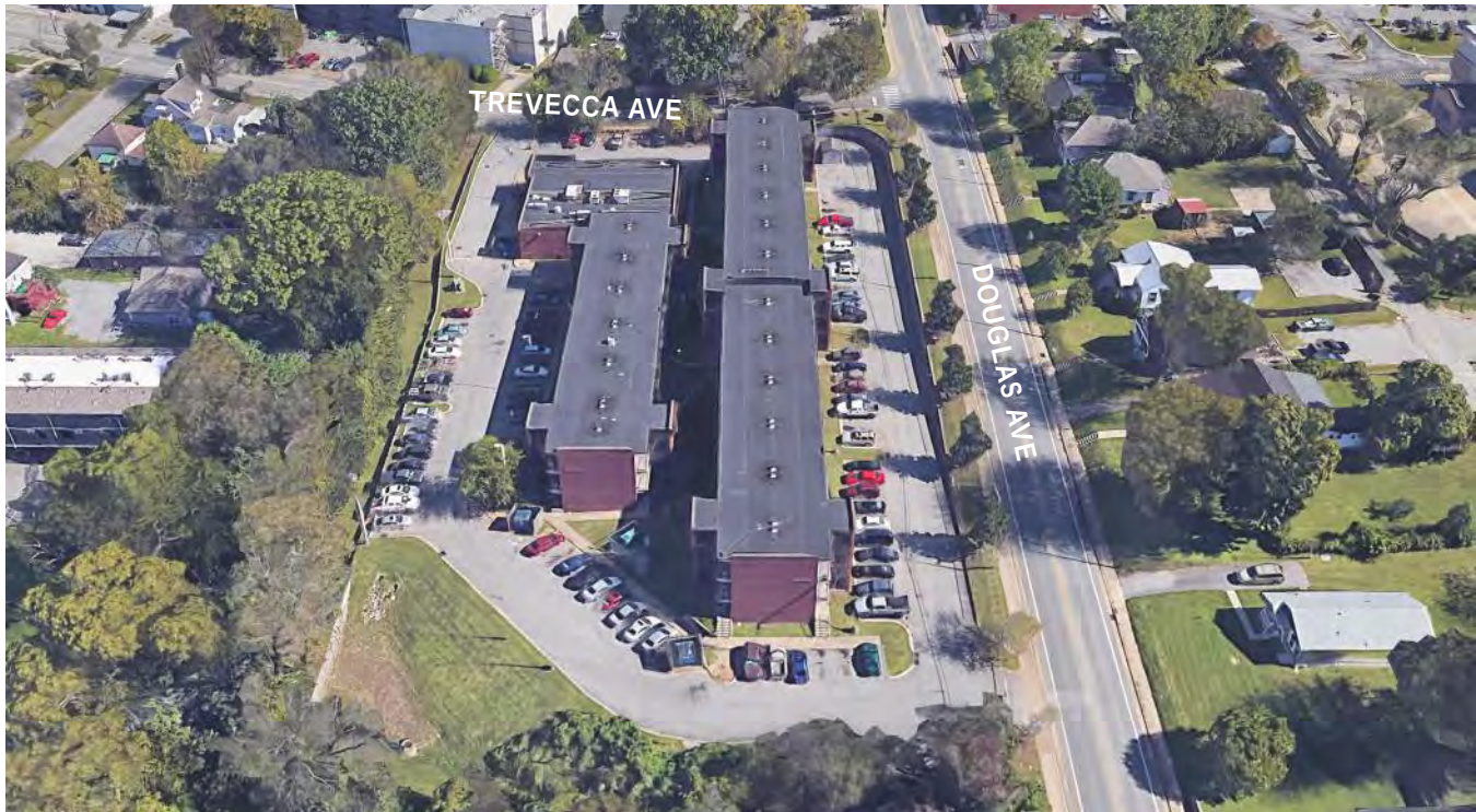
BIRD'S EYE VIEW LOOKING EAST
