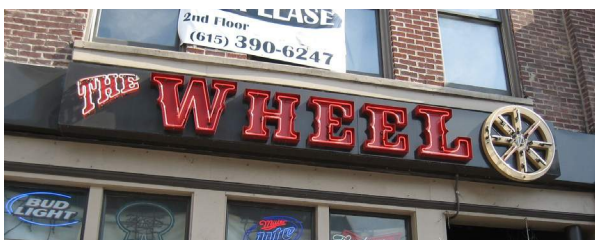
Example of raceway incorporated as sign background
