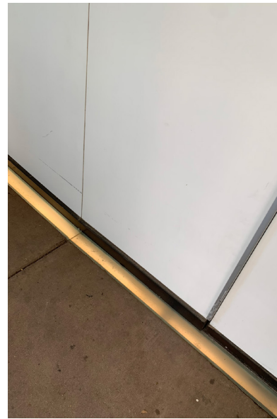
EXISTING LIGHTING FIXTURE
