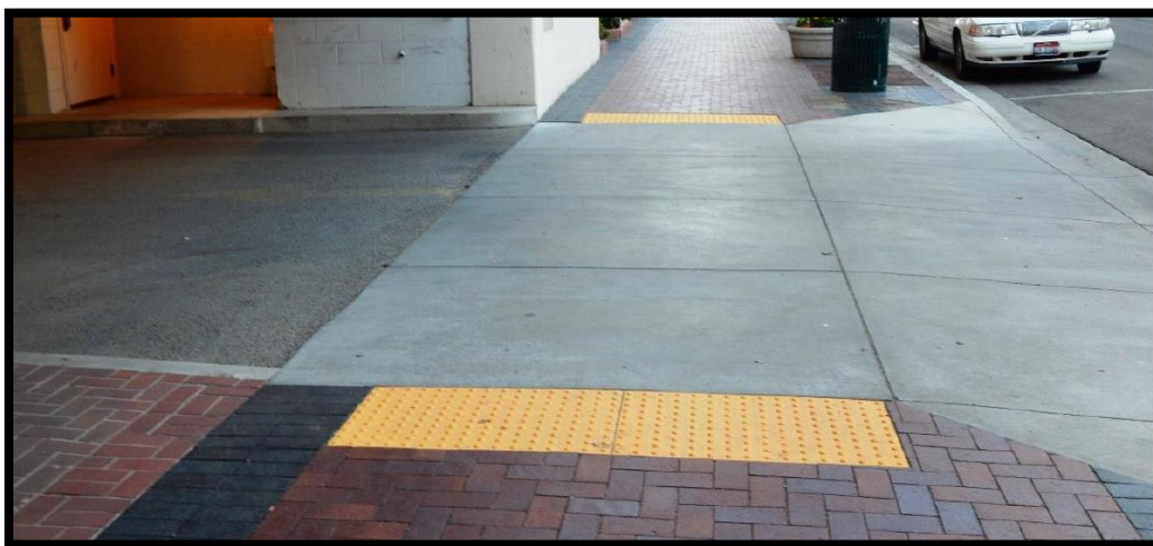
Figure 4-7: Garage Access Ramp Flush with Sidewalk
