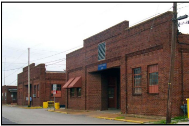
WPA Municipal Garage
