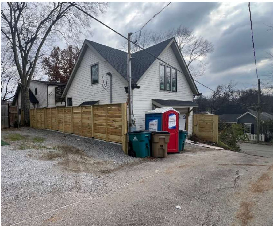
SITE AS SEEN FROM IMPROVED ALLEY
