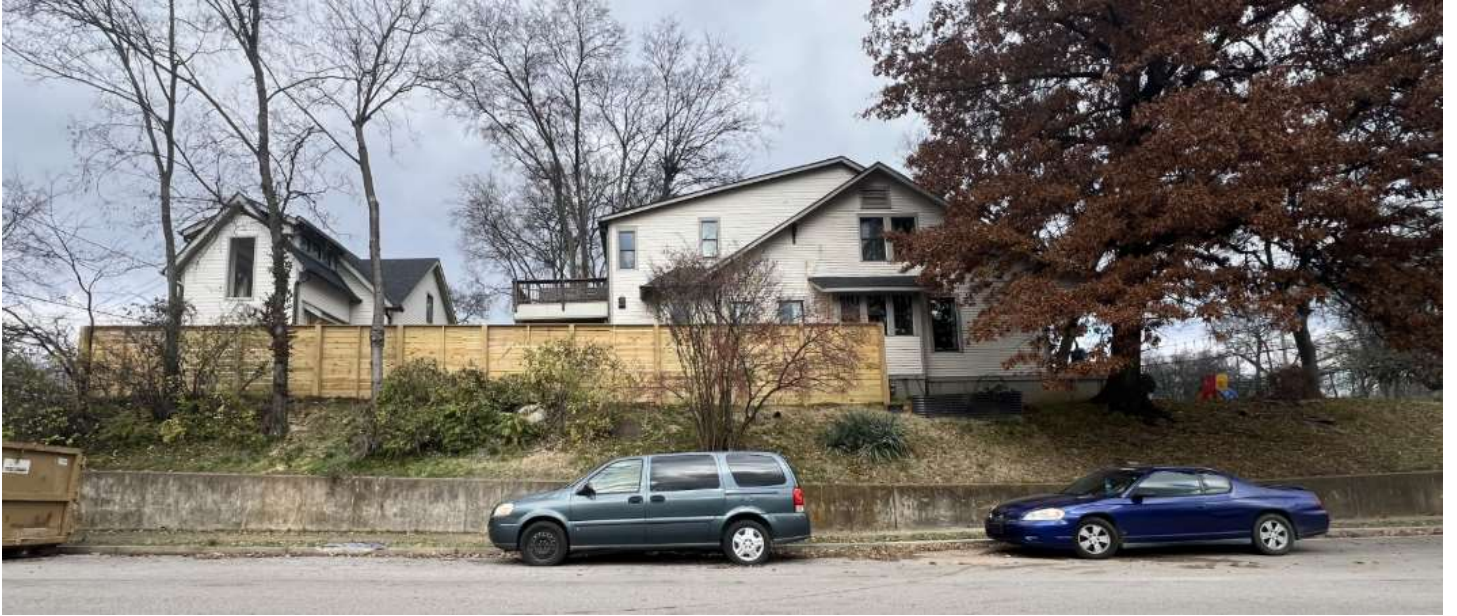
SITE AS SEEN FROM MARINA STREET
