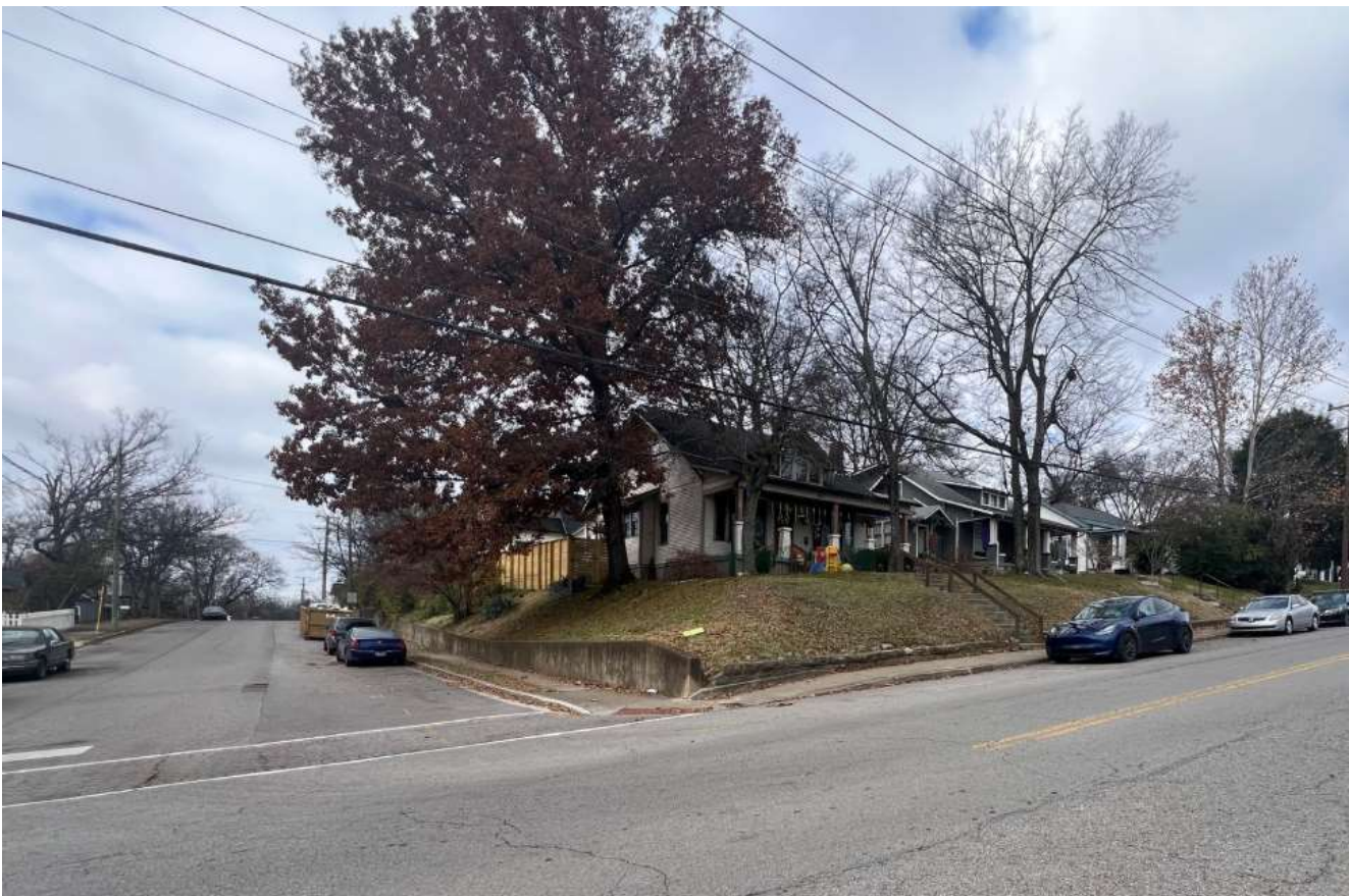
SITE AS SEEN FROM MCFERRIN AVENUE
