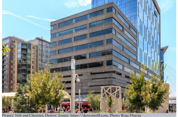
Project: 16th and Chestnut, Denver. Source: https://denverinfill.com , Photo: Ryan Dravitz
