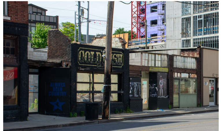
Doors and windows were replaced prior to designation but the dimension and design of entries should be retained.
