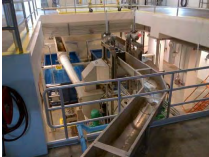
Figure 3-5. Example of a sluice channel (uncovered) discharging to a pair of screenings compactors
