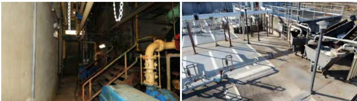
Figure 14-1. Existing Grit Tank Tunnel and Upper Level Photos
