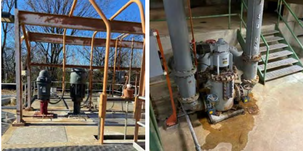
Figure 14-5. Existing HPE Pumps (L) and Strainers (R) to be demolished.
