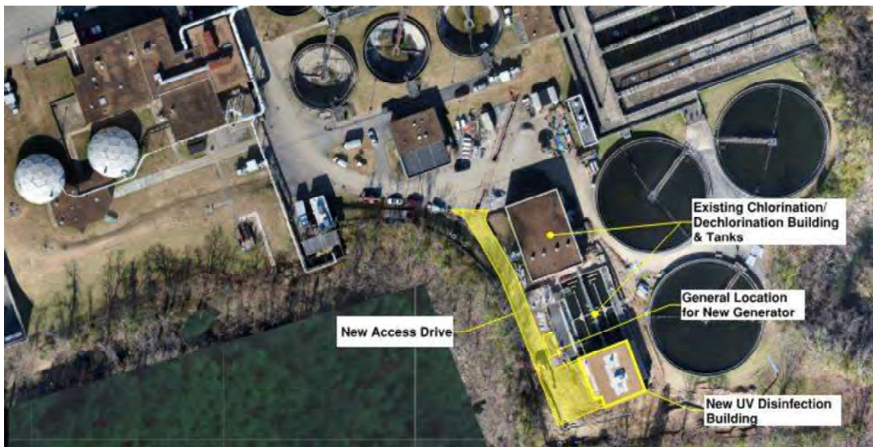
Figure 1-3. December 2021 Aerial Photograph with New Facilities Highlighted
