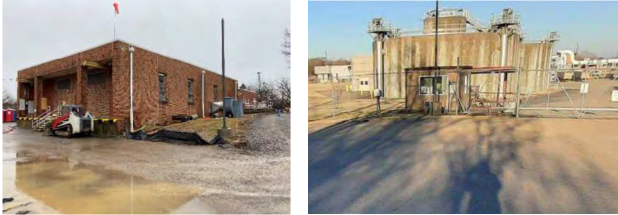
Figure 14-9. Chlorination Building (L) and Security Guard Booth (R) to be demolished
