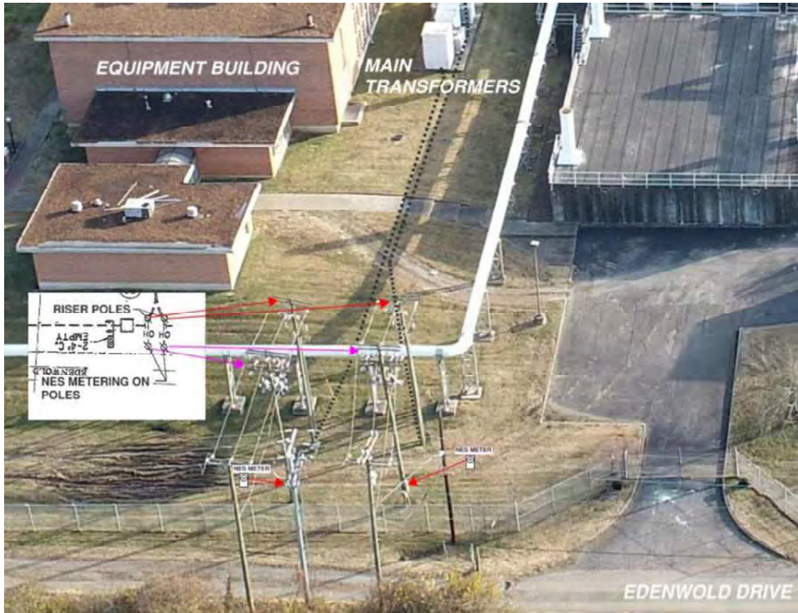
Figure 11-1. NES Service Arrangement
