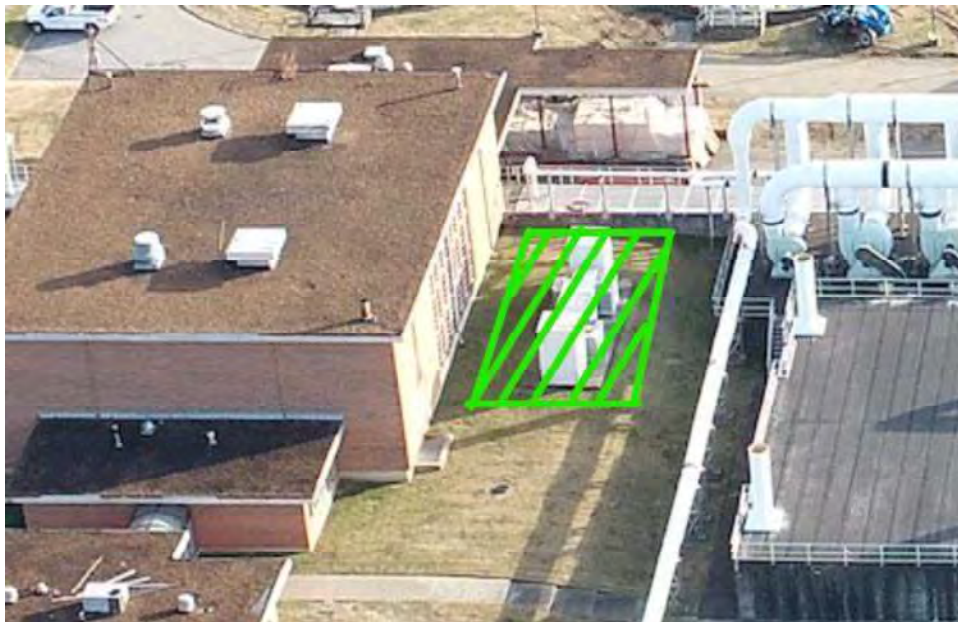
Figure 14-4. MV Switchgear Demolition
