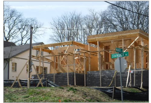
New construction in progress on Stainback Avenue
