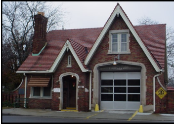
21st Avenue South Firehall
