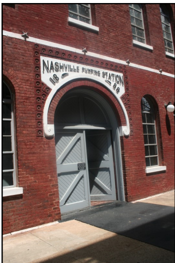
Omohundro Water System
