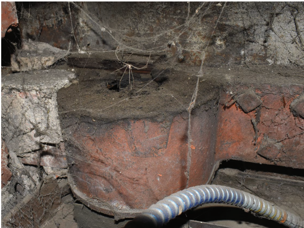
Detail image of the header hinge above the entryway ceiling. Image by TTG.
