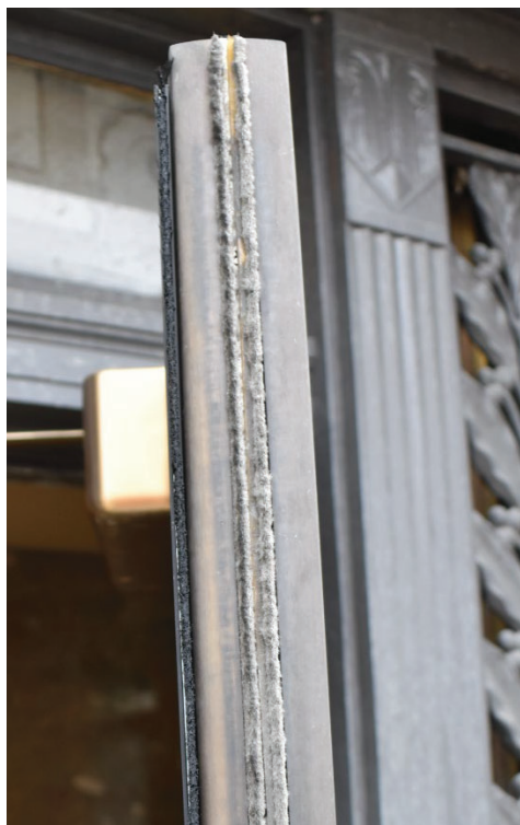
Detail images (at left and above) of weather stripping types. Images by TTG.
