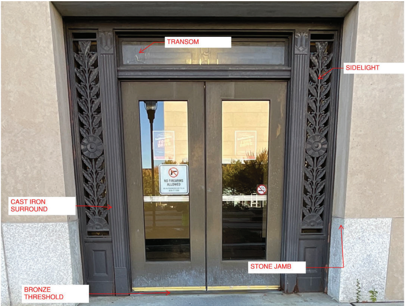
Elevation image of the typical doors found on the north façade of the courthouse. Image by TTG.
