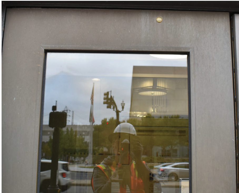
Detail image of a typical door exterior cladding on the north façade of the courthouse. Image by TTG.
