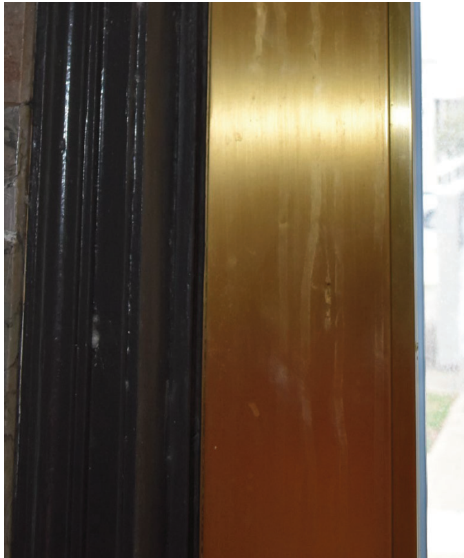
Detail image of the door cladding found on the interior of the west elevation doors. Image by TTG.
