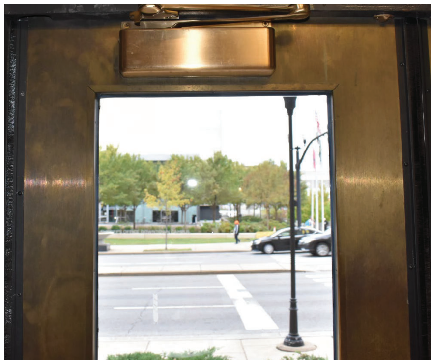
Detail image of a typical door interior cladding on the north façade of the courthouse. Image by TTG.
