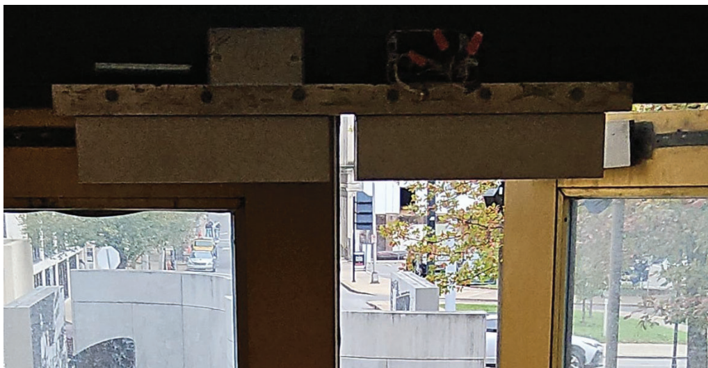
Detail image of the magnetic closer present on the west façade doors. Image by TTG.
