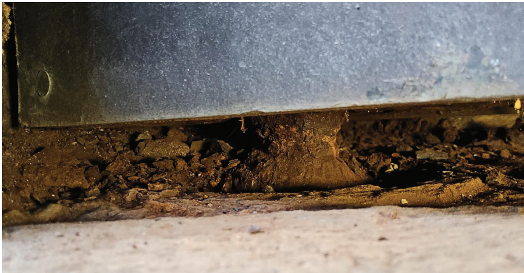
Detail image of the severely deteriorated hinge pin observed during the assessment. Image by TTG.
