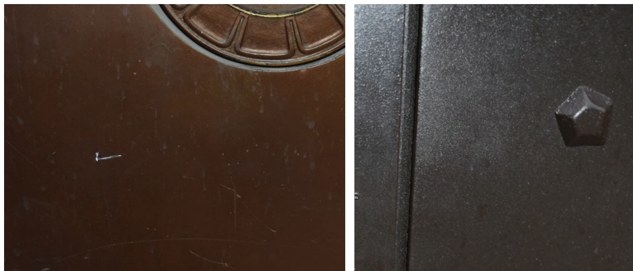
Detail images of the faux bronze patina applied to the surfaces of the bronze doors. Images by TTG.
