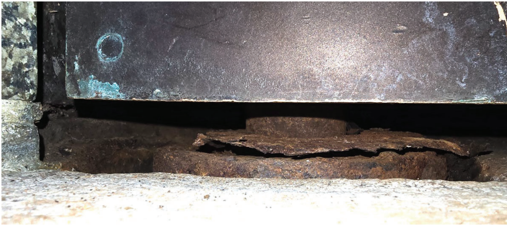
Detail image of the threshold hinge body embedded in the stone threshold. Image by TTG.
