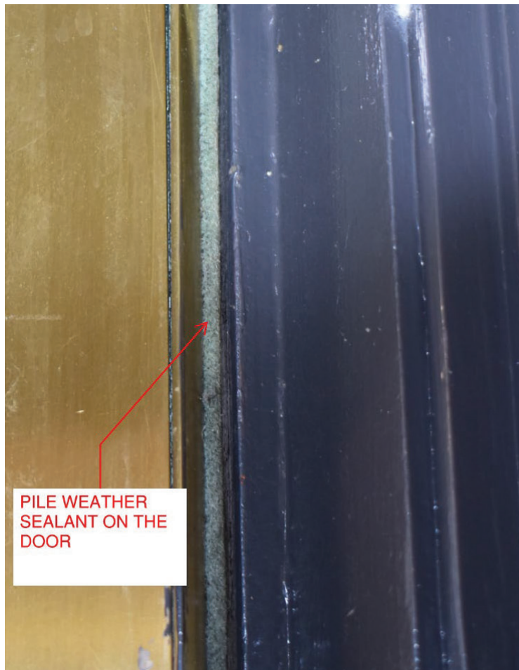
Detail image of pile weather sealant. Image by TTG.
