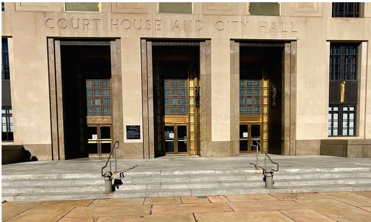
Elevation image of the three pairs of bronze doors found on the south façade of the courthouse. Image by TTG.
