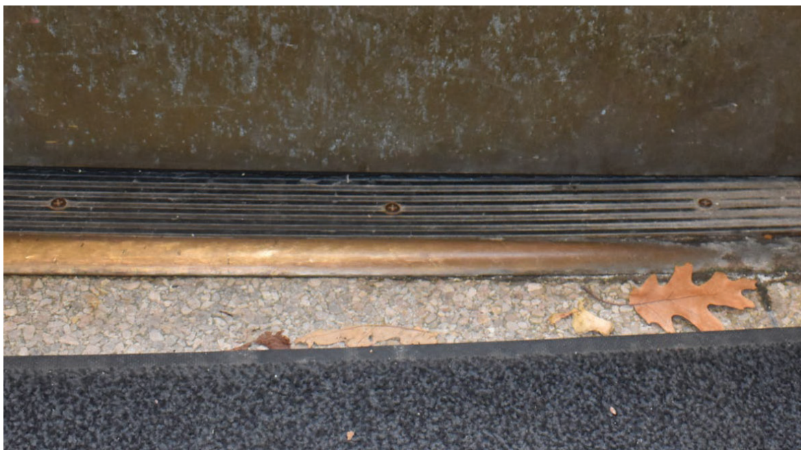
Detail image of a typical threshold found on the north façade doors of the courthouse. Image by TTG.
