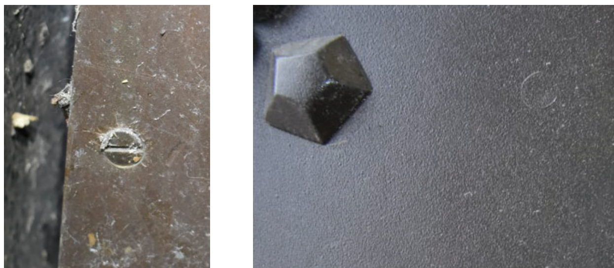
Detail images of the interior side of the cladding fastener (at left) and the exterior side of the cladding fastener (at right). Images by TTG.
