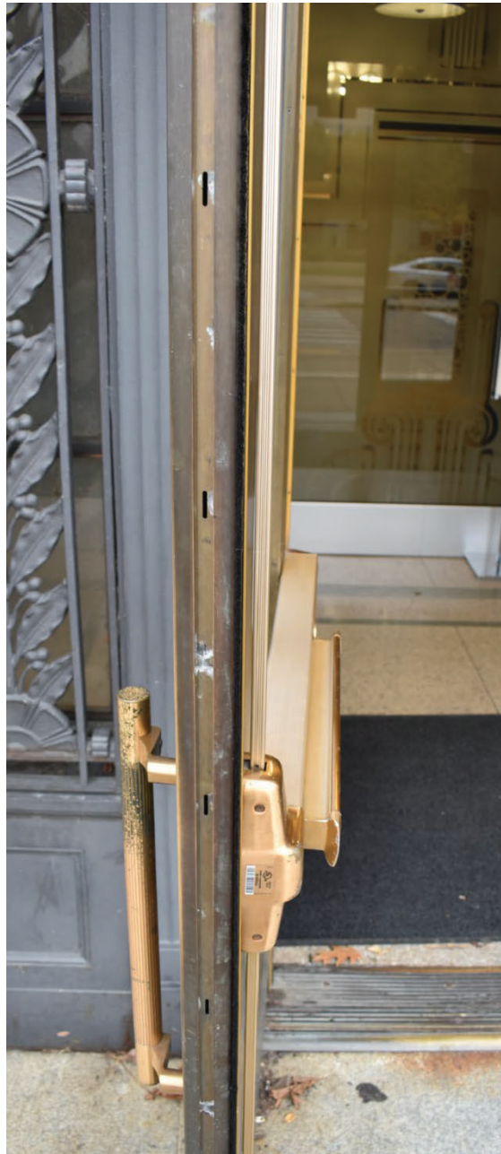
Detail image of weather-stripping on north façade doors. Image by TTG.
