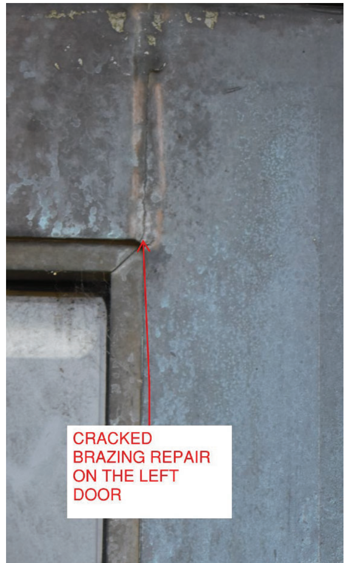
Detail images of various previous repairs and failure at the door rails. Images by TTG.
