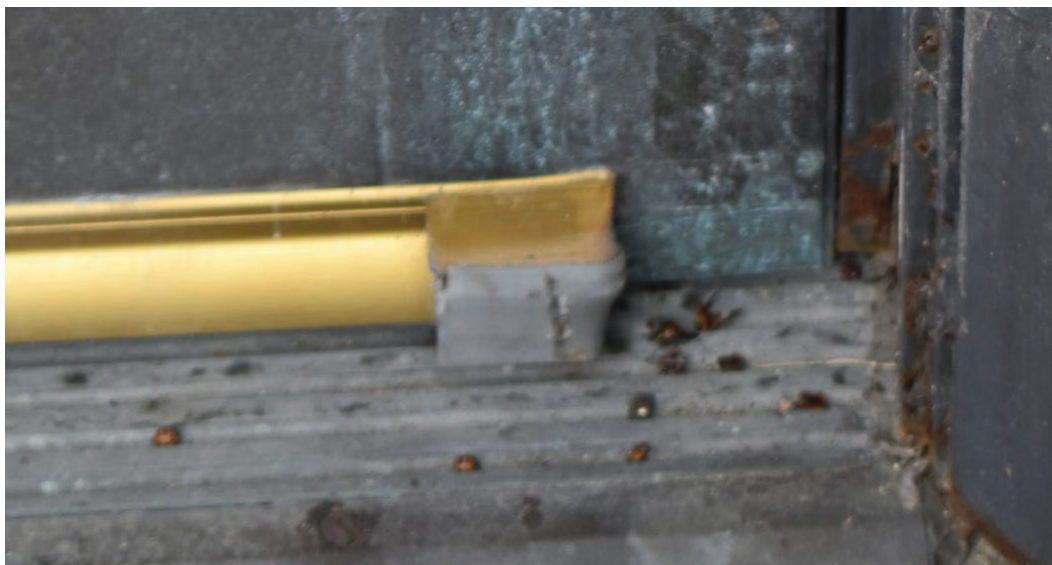
Detail image of folded weather stripping. Image by TTG.
