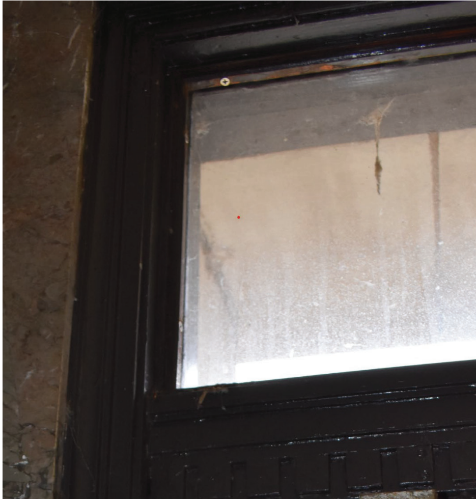
Detail image of the transom above the doors found on the west façade. Image by TTG.
