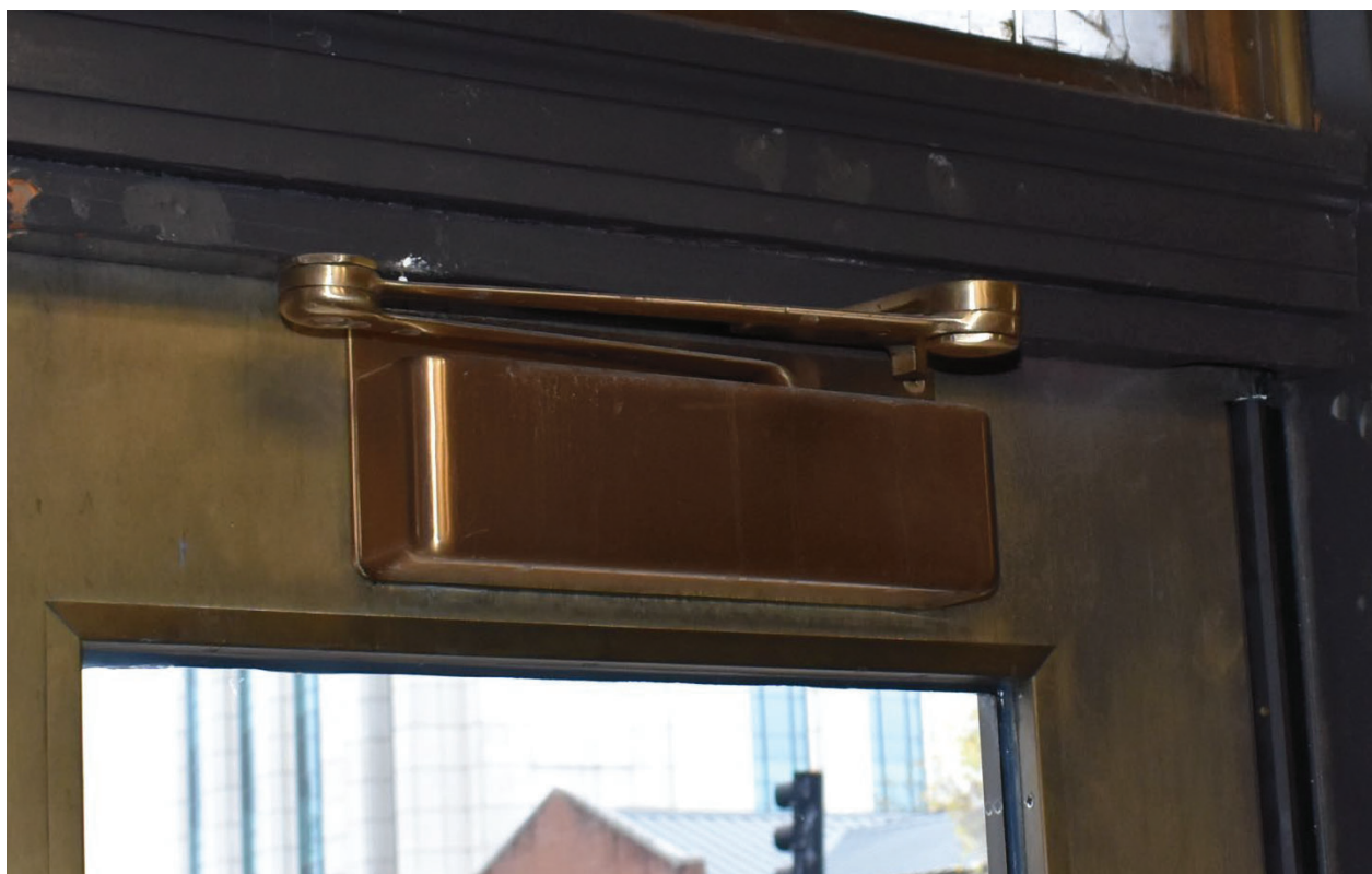
Detail image of the brass finished door closer. Image by TTG.
