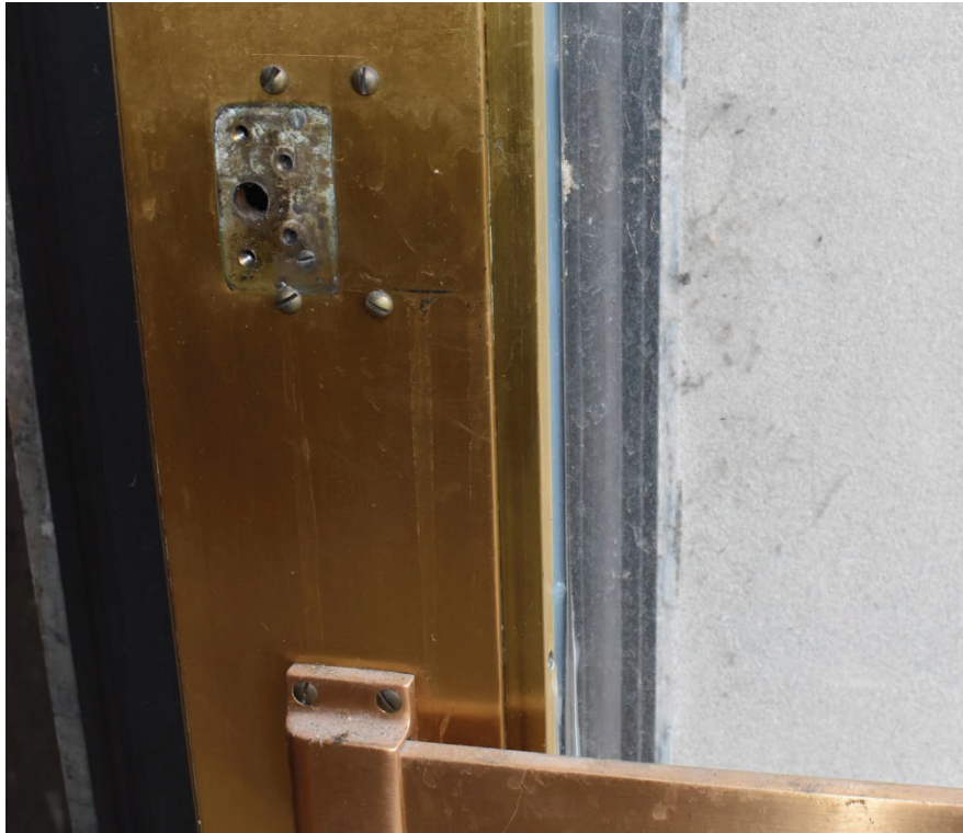
Detail image of remnants from previously installed hardware. Image by TTG.
