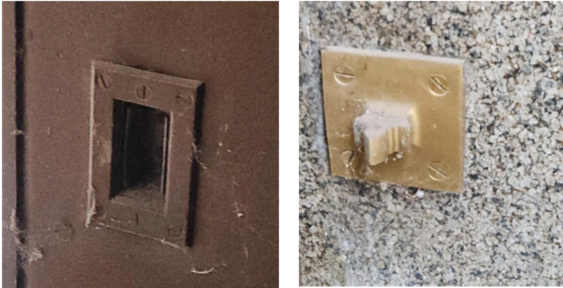
Detail images of the door catch receiver (at left) and the bronze door catch (at right). Images by TTG.
