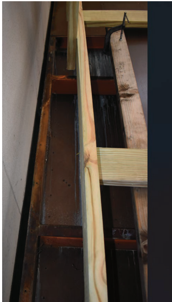
Detail image of the subframe of the bronze door. Image by TTG.
