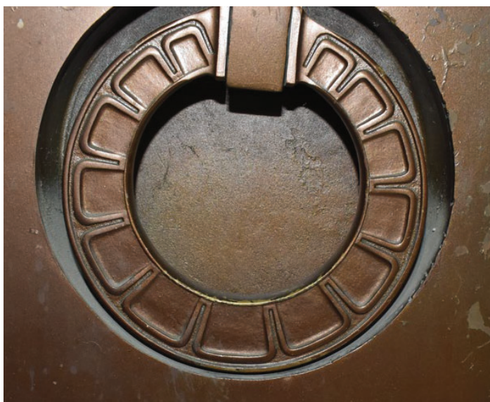
Detail image of the typical round hinged door pull inset into the back of the bronze doors. Image by TTG.
