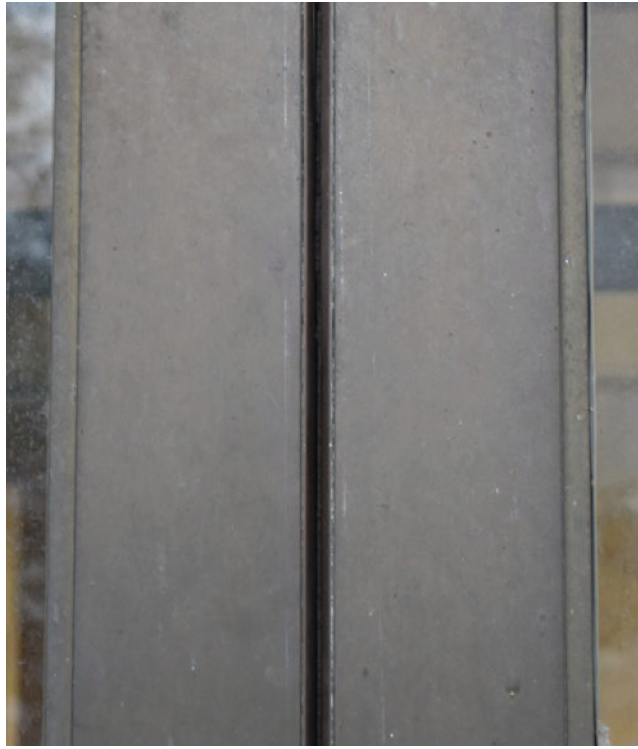
Detail image of the door cladding found on the west elevation doors. Image by TTG.
