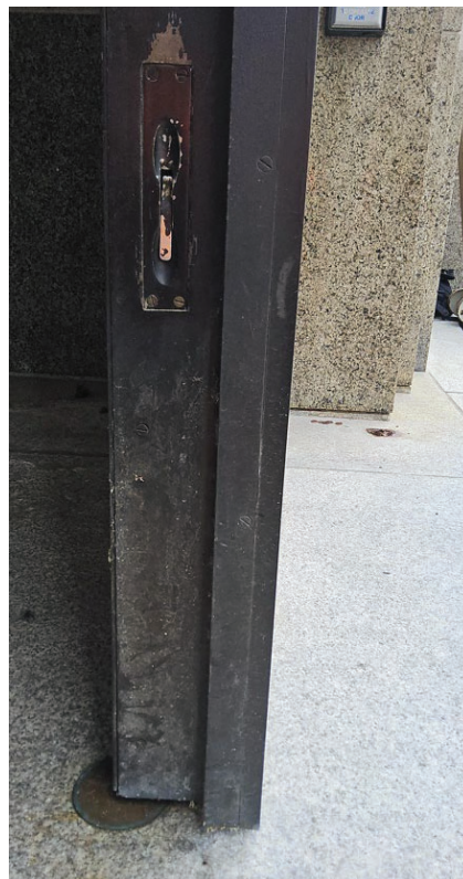
Detail image of the threshold and header security bolt. Image by TTG.
