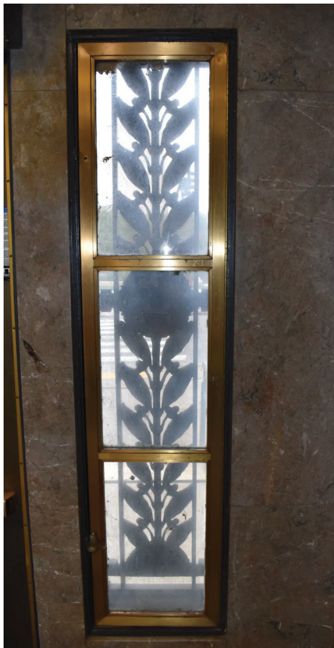
Detail image of the interior side of a typical sidelight found on the north façade doors. Image by TTG.
