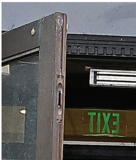
Detail image of the multilayered bronze door assembly. Image by TTG.
