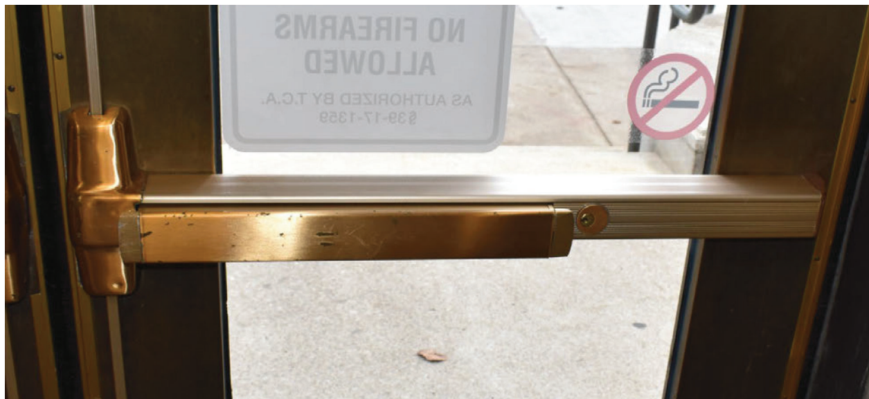
Detail image of a push bar on the interior side of the door. Image by TTG.
