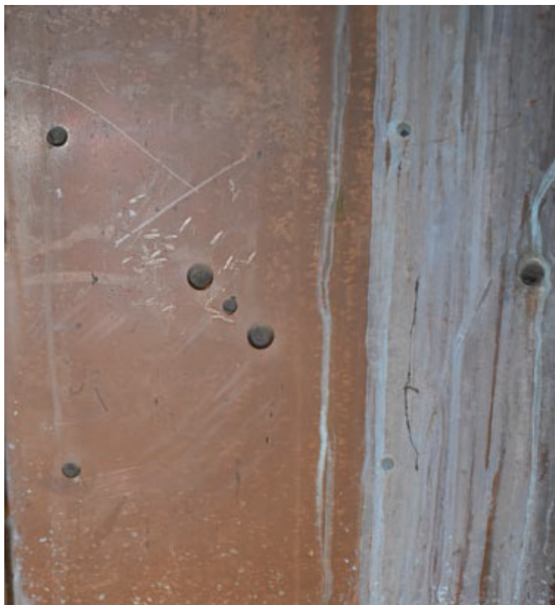
Detail image of the rivets that secure the statuary and decorative elements to the bronze cladding. Image by TTG.
