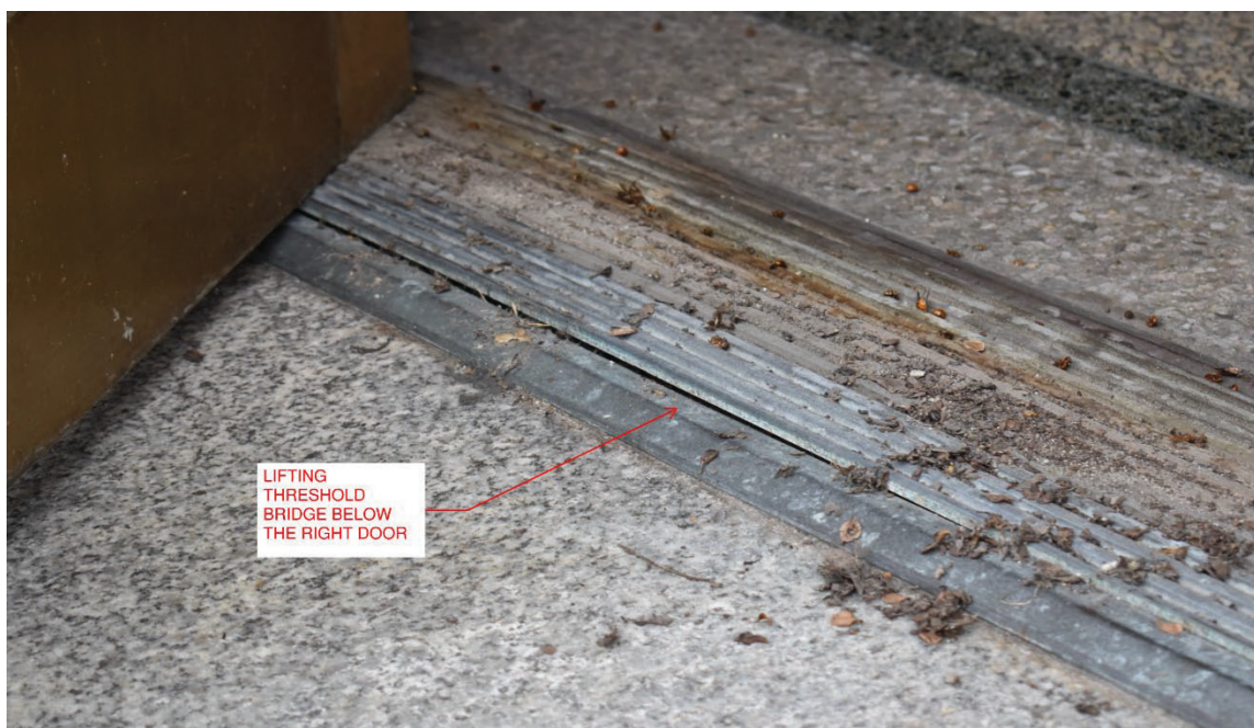
Detail of lifting threshold. Image by TTG.
