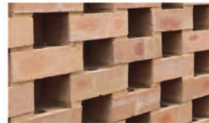
Brick walls with perforation
