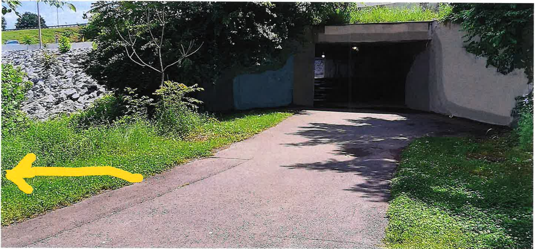
Looking East on Stones River Greenway to tunnel under S.R. 155 from beginning point of Opry Mills Greenway Connector. Pedestrian Bridge to west.
