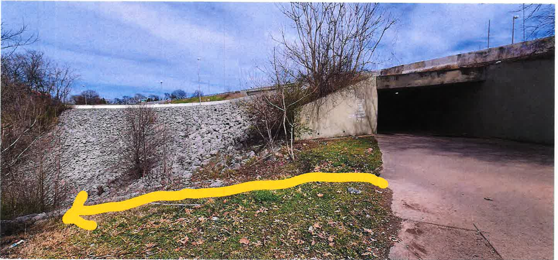
Looking towards tunnel in winter season.
