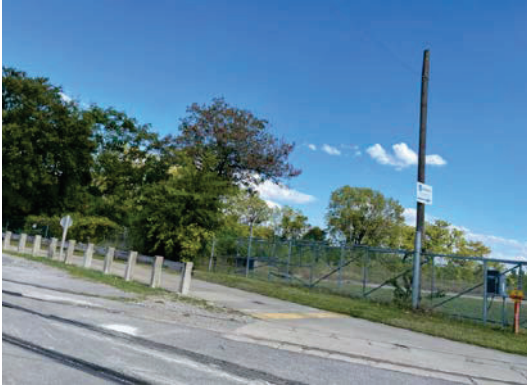
Cement Plant Road facing East
