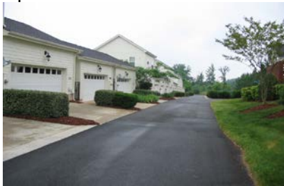
Parking garages accessed from rear
