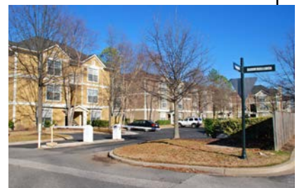
Landscaping and screening
