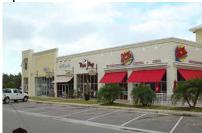
One row of parking in front of building
