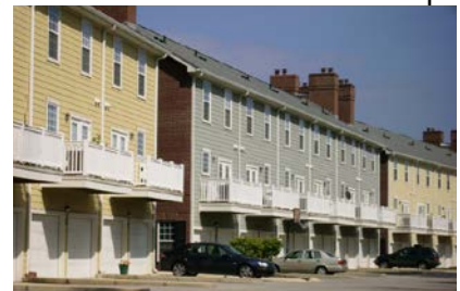
Rear access parking garages
