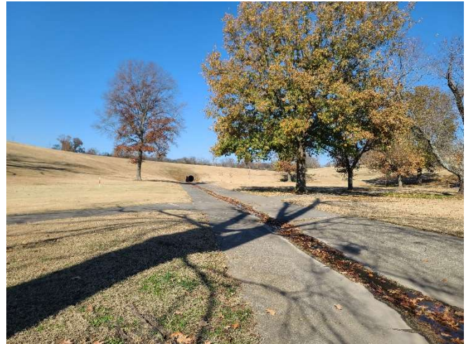
PRP 3 - Looking Upstream at oversized concrete channel on UT1 Reach 1
