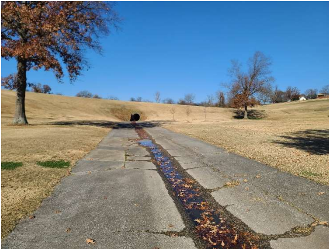
PRP 2 - Looking Upstream at oversized concrete channel on UT1 Reach 1
