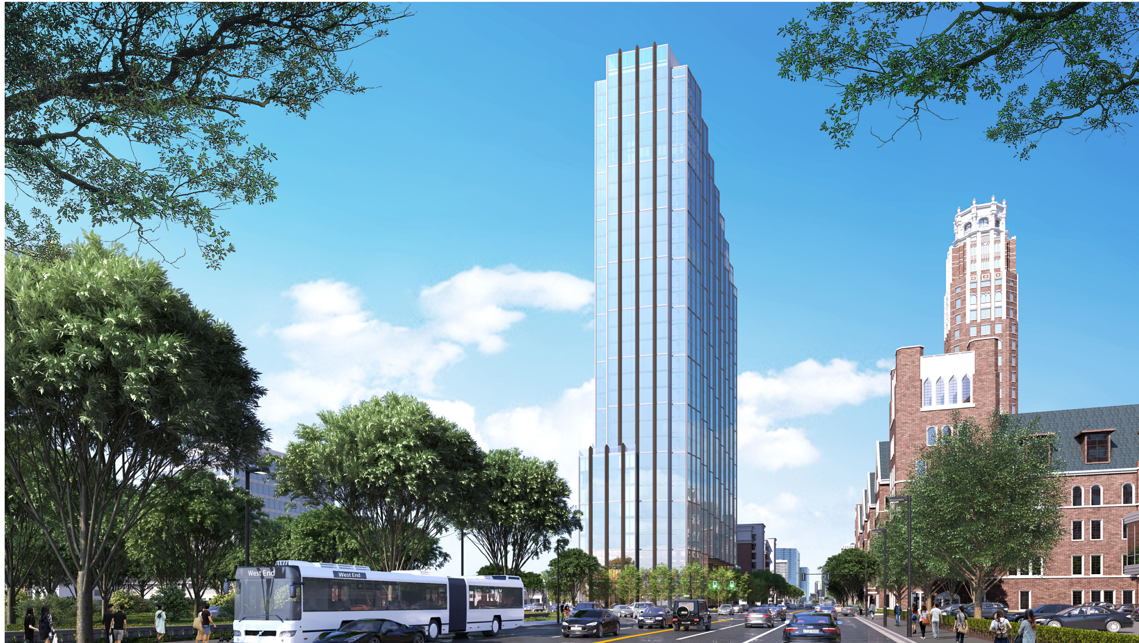
VIEW FROM WEST END LOOKING EAST
