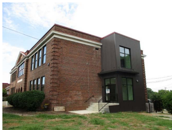
Side of Improvement/Recent Addition
