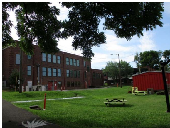
Rear of Improvement
