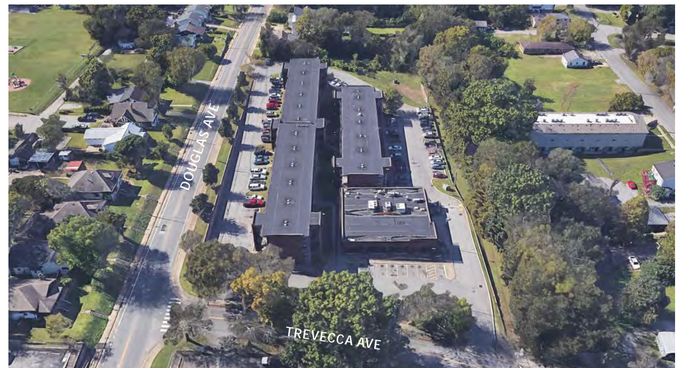
BIRD'S EYE VIEW LOOKING WEST
