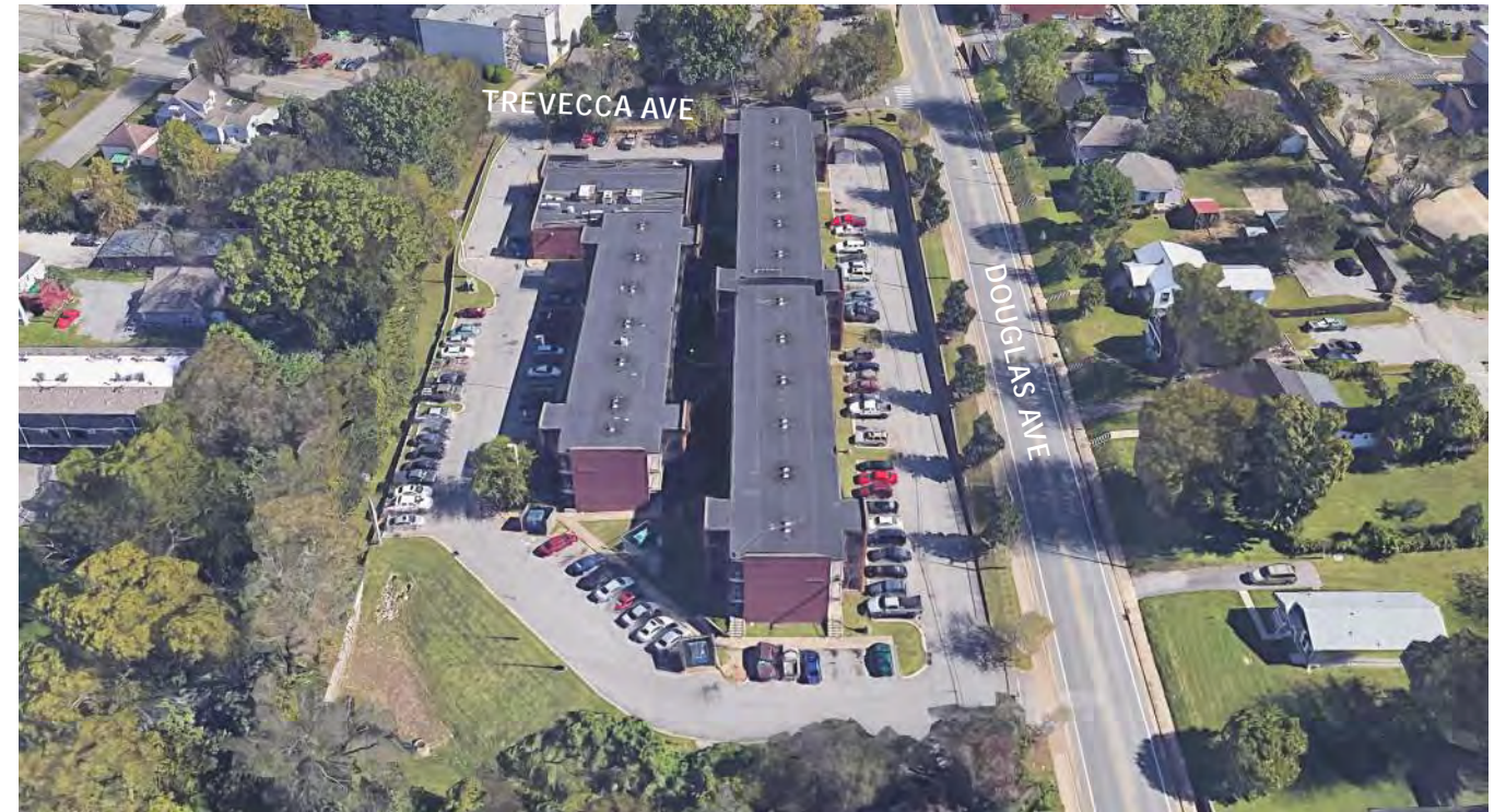
BIRD'S EYE VIEW LOOKING EAST
