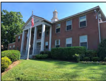
James A. Cayce Administration Service Building
