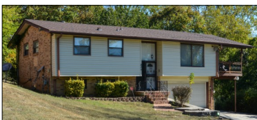
825 Youngs Lane is an example a cantilevered second level.
