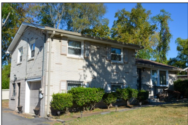
Split Level house at 1906 Lathan Court.
