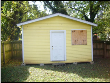
Example of a small storage building without a permanent foundation.
