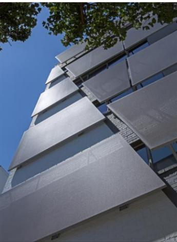
Dark tensile background pattern with lighter raised pattern and accent color. Modular panels with steel clips
