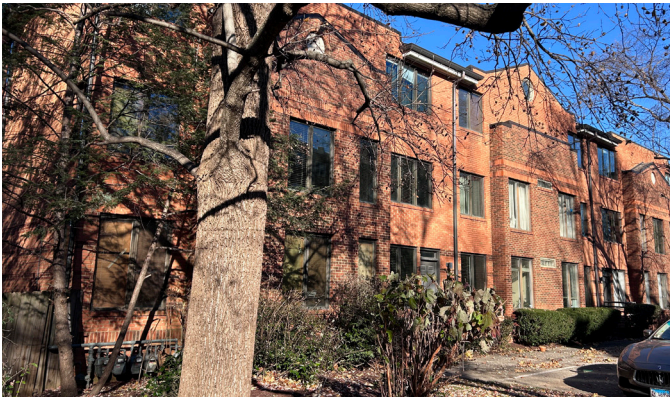
Multiplex with a recessed stoop entry.
