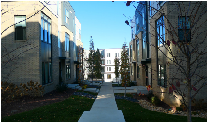
Townhouse Court along a pedestrian passage.
