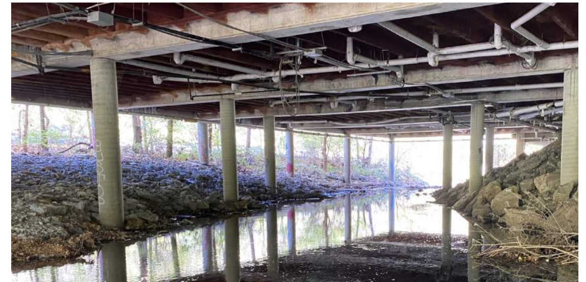
1. EXISTING CREEK CONDITION UNDER THE GROCERY STRUCTURE
