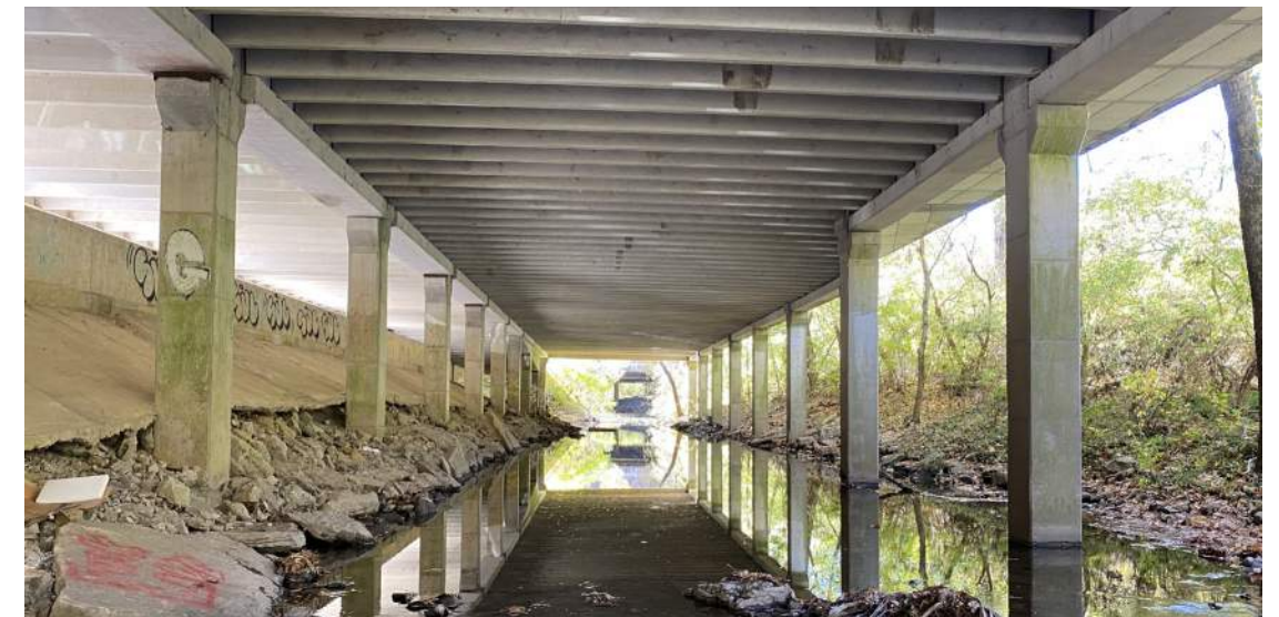
2. EXISTING CREEK CONDITION UNDER THE PARKING STRUCTURE
